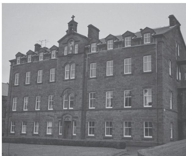
St Joseph's College rear building, Dumfries, 1982 (SC 1876133 © Crown Copyright: HES).
