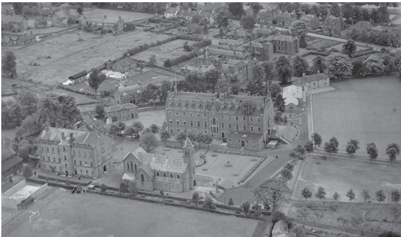
Aerial photograph of St Joseph's College, Dumfries, 1939 (SC 1438729 © Crown Copyright: HES).
